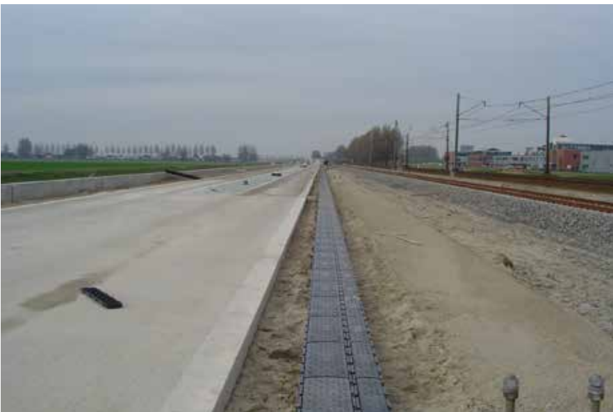
Example of a cable duct installation in Netherlands
